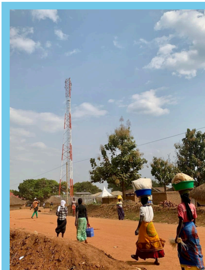
Infrastructure in Yumbe, Uganda.
